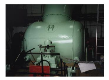
Hydro-Electricity production was restarted after restoration of the mill lade and the 1930s turbine in Mill No.3
