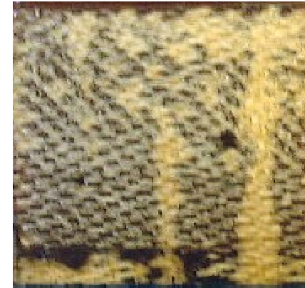
Surface failure (epoxy)
