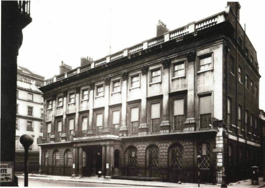
The bank in 1942 with sticky tape on the windows to protect the glass from bomb blast.
