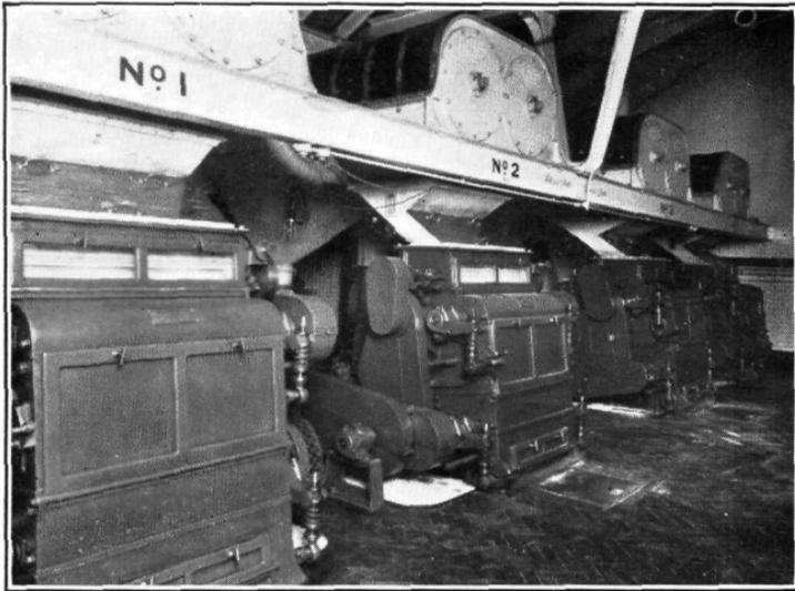
*THE MILLS USED FOR GRINDING THE MALT*
