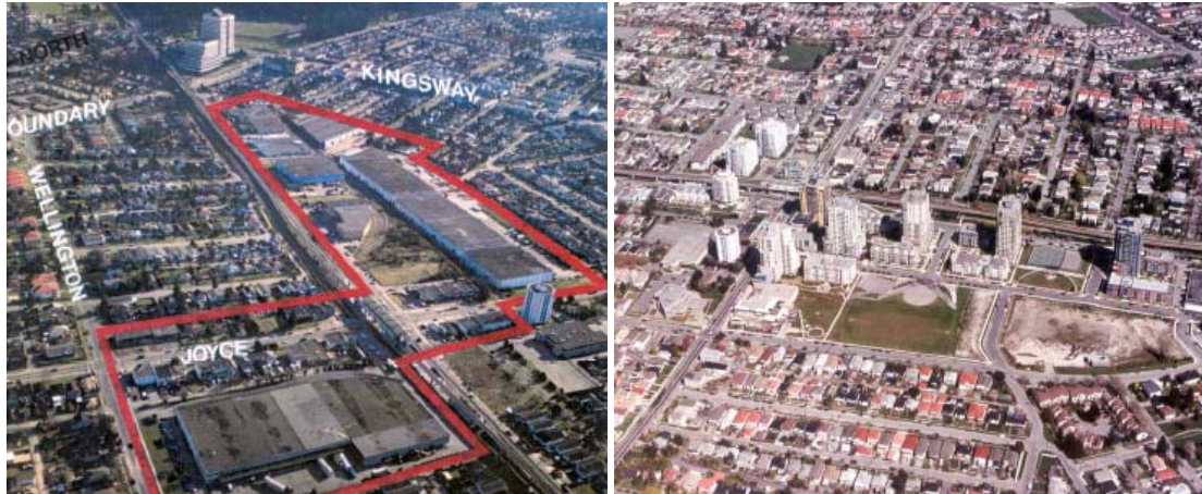
Figure 8: Collingwood Village at Joyce Station: Before and After (1993-2000) – A Model North American PTOD (Concert Properties)
